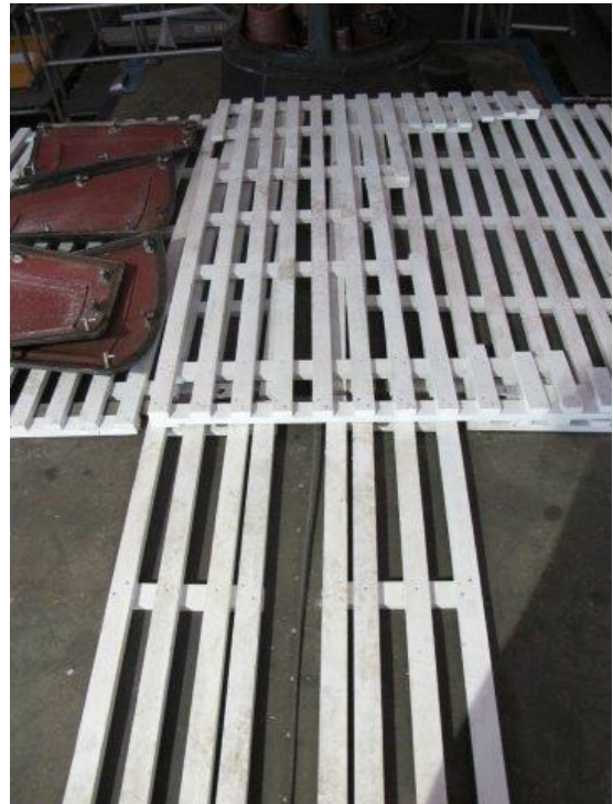
Type 86 cabin roof with decking being replaced
